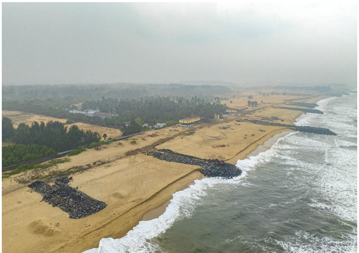
After Placing Groynes
