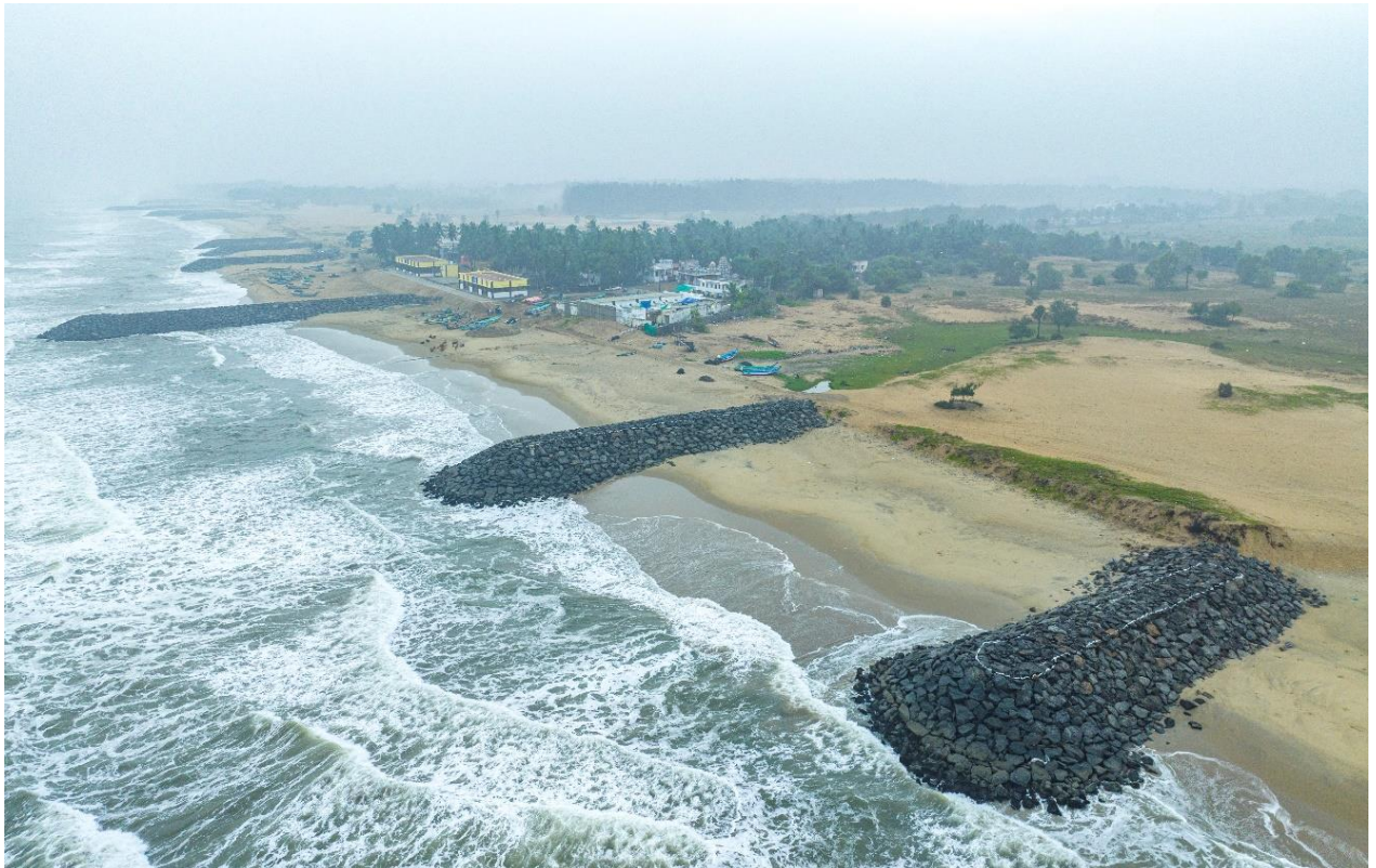
After Placing Groynes
