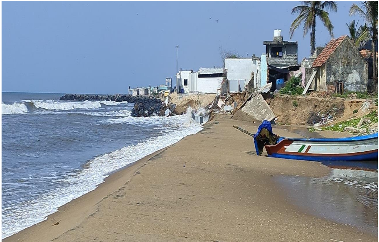
Before Placing Groynes
