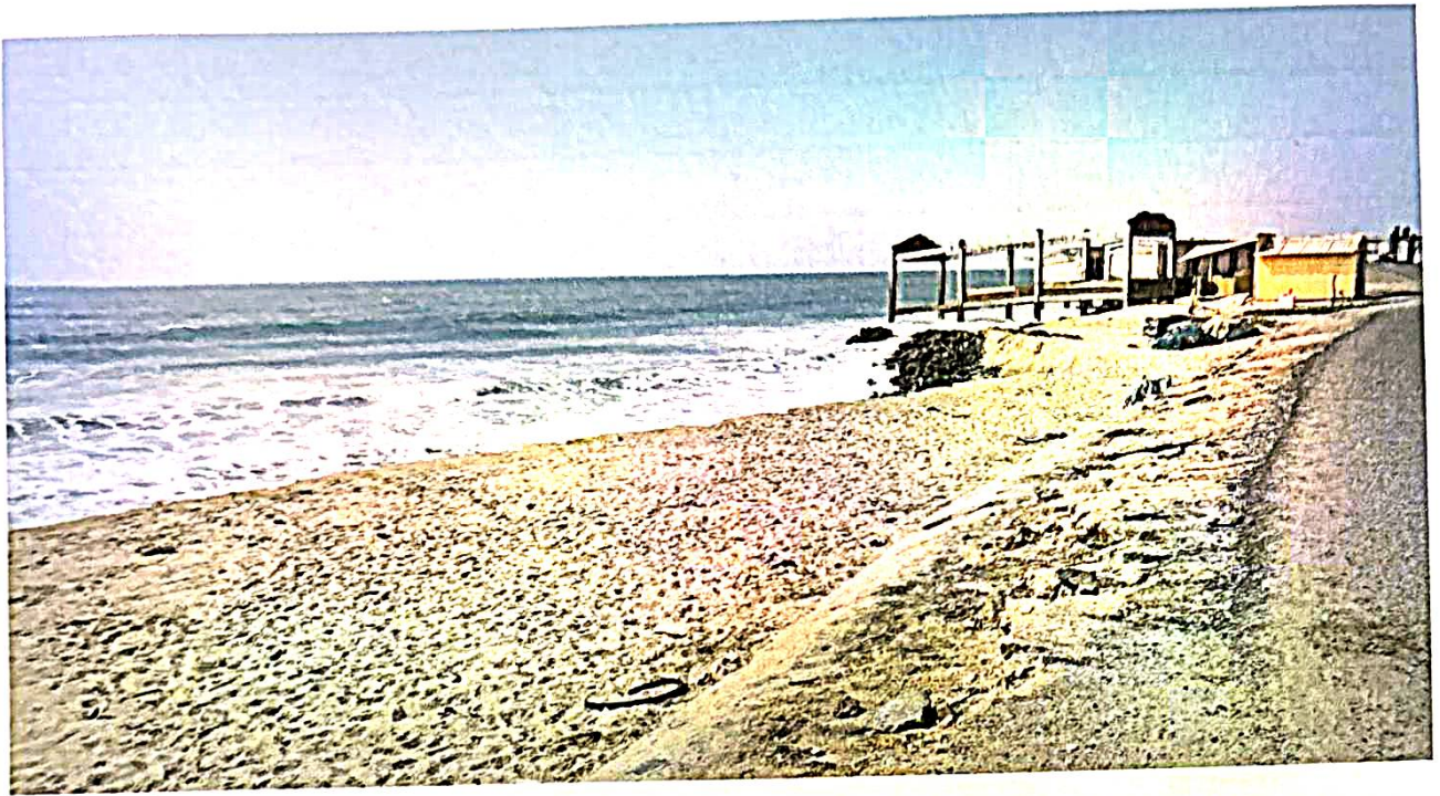
Kadalore Periyakuppam Beach and building eroded photos
