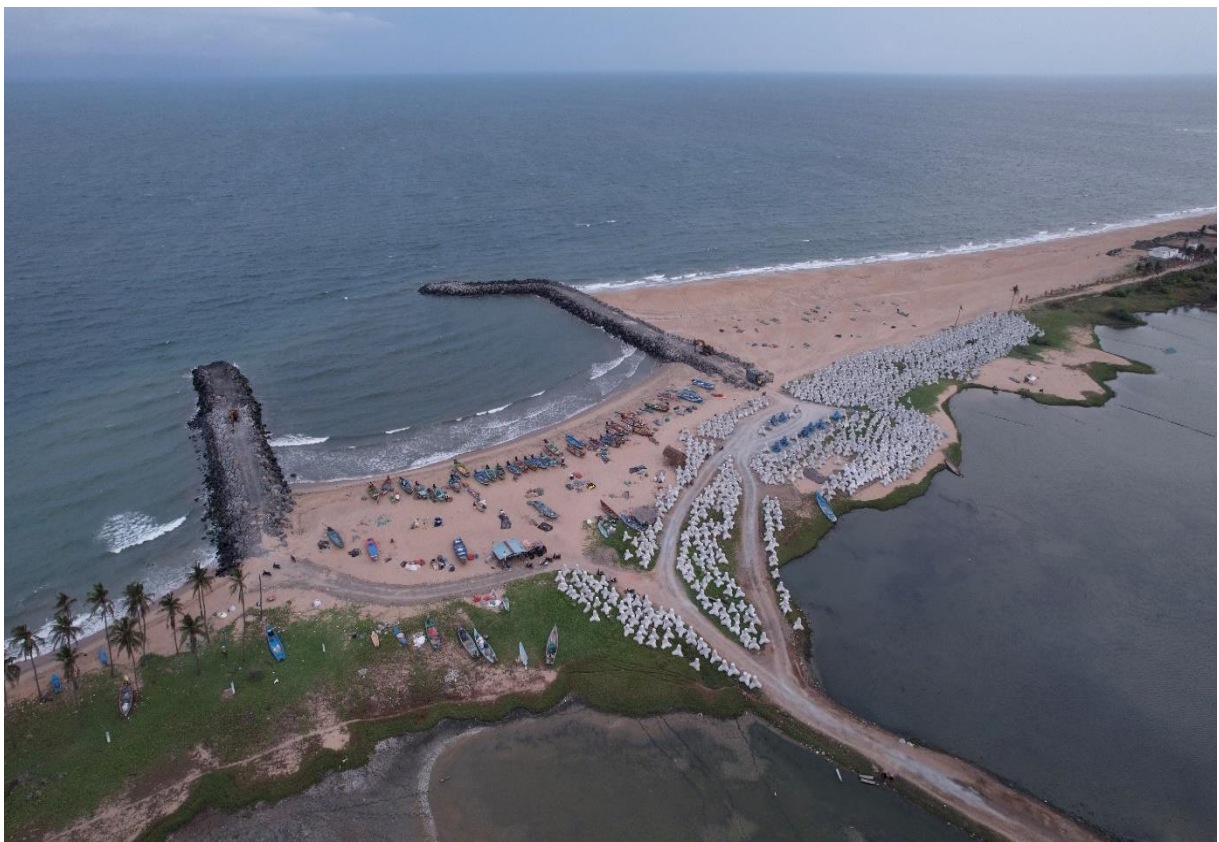
After Placing Breakwaters
