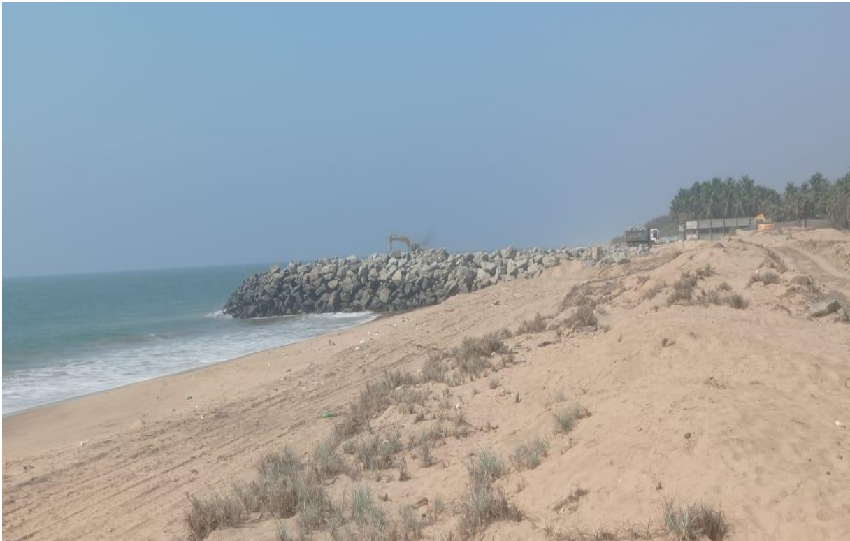
During Execution of work
