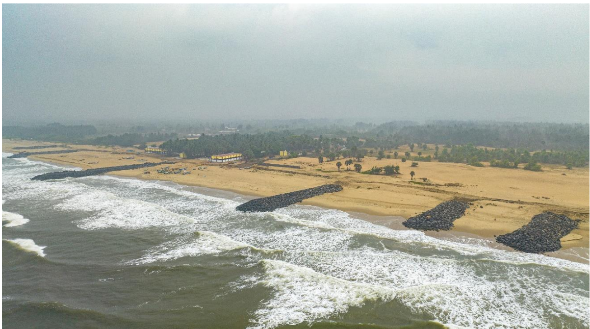
After Placing Groynes
