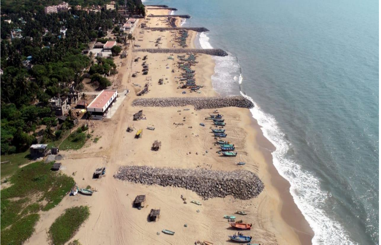
After Placing Groynes
