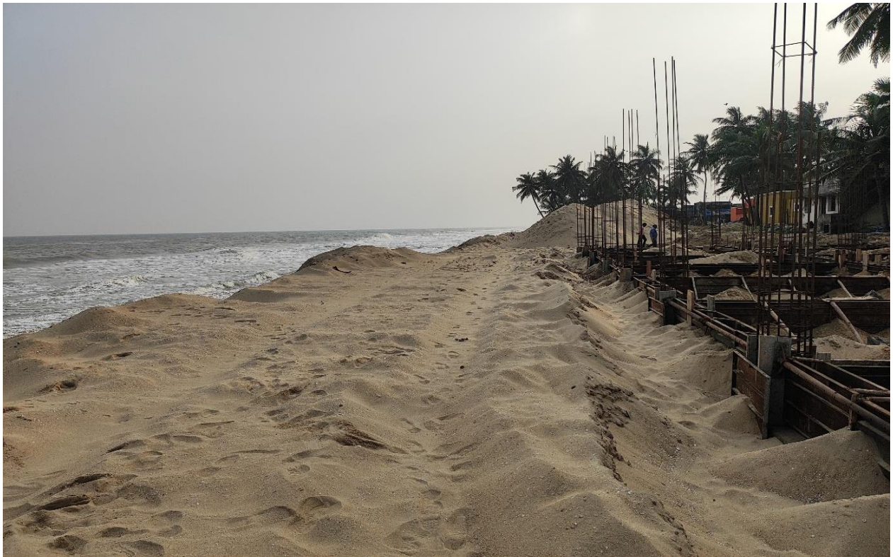
Before Placing Groynes
